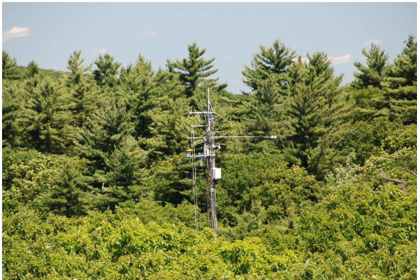
Figure 1: The EMS Tower as viewed from Walkup.
