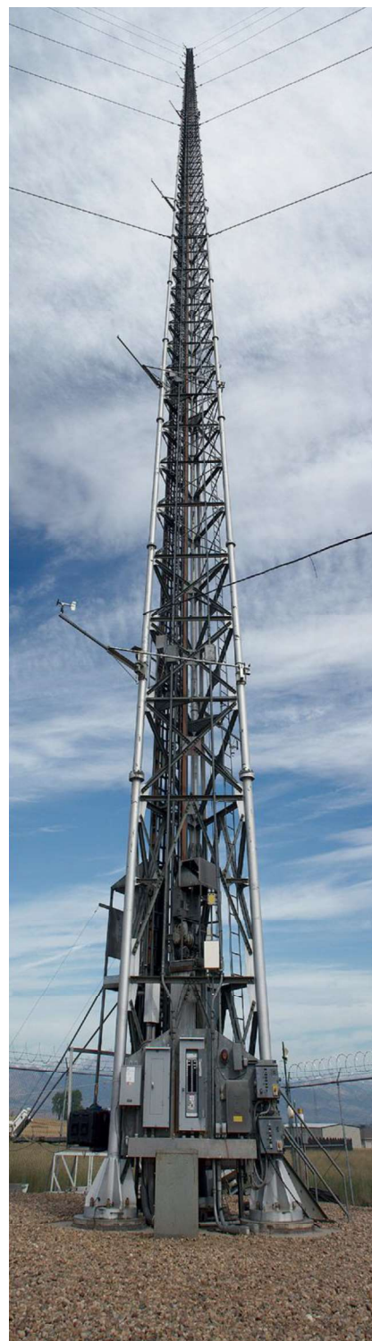
FIG. 1. The southeast face of the 300-m Boulder Atmospheric Observatory (Photograph courtesy of Dr. Shelby Frisch).
